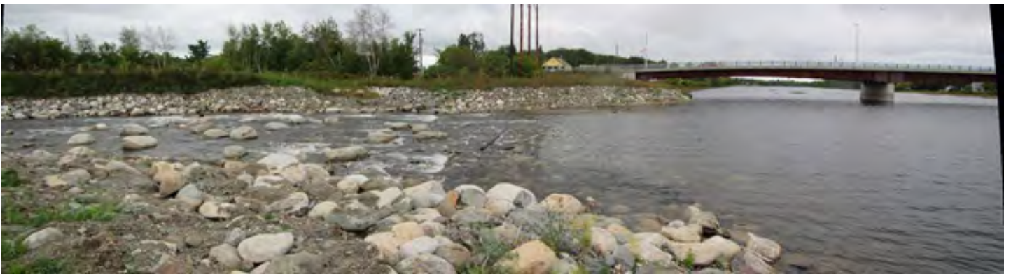
Top: Upstream entrance to the Howland bypass channel. Right: Boulders placed in the bypass channel.
