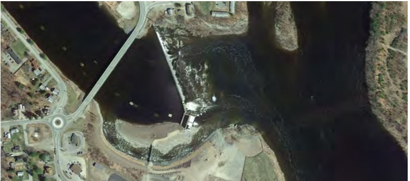
Completed Howland Bypass Channel on the Piscataquis River, tributary to the Penobscot River, ME (right side of picture).
