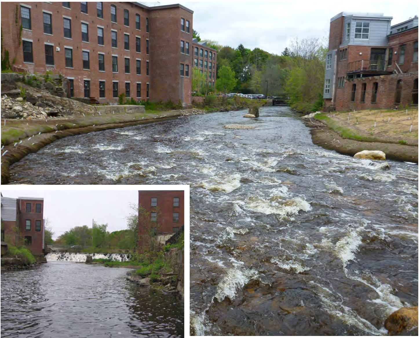
Top: After removal of the Marland Place Dam and construction of riffles. Bottom: Marland Place Dam before removal.
