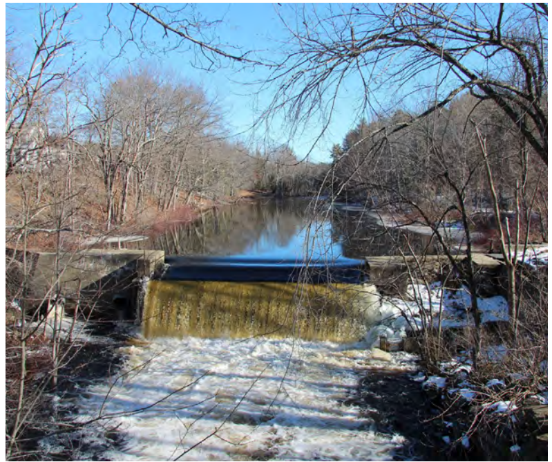
Coopers Mill Dam.
