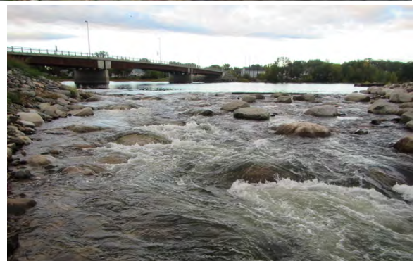
Top: Upstream entrance to the Howland bypass channel. Right: Boulders placed in the bypass channel.
